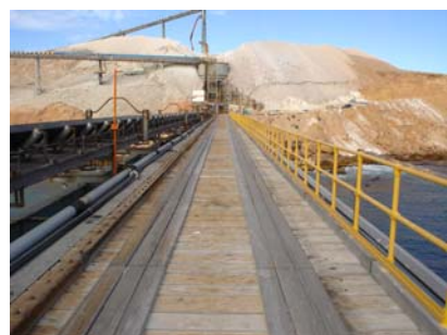
Handrails at Dampier Salt site
